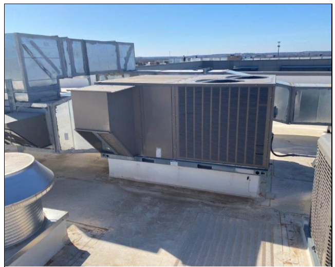
66. Packaged unit at roof
