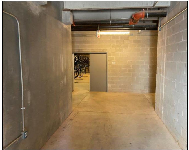
28. Concrete slab-on-grade with concrete foundation walls
