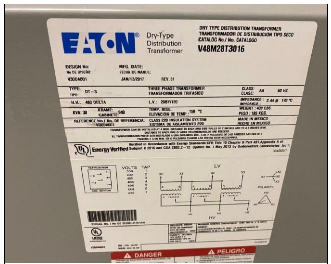
72. Step down transformer label
