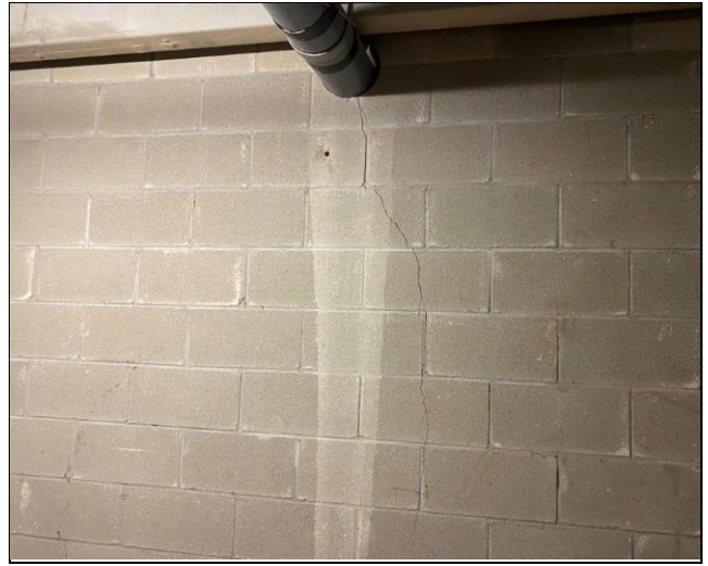
104. Linear cracking of load bearing CMU block walls at the bottom level
