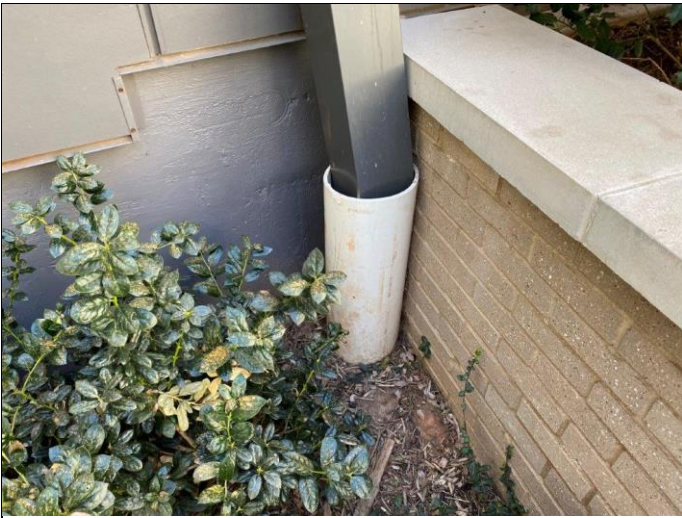
3. Downspout at courtyard draining directly into the storm sewer system, typical
