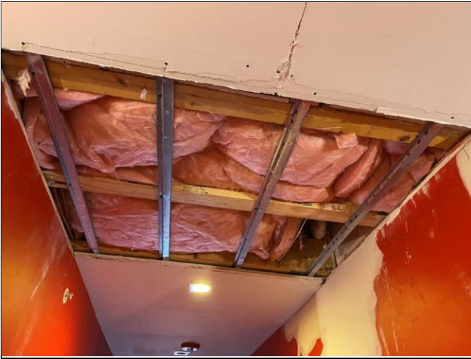
31. Wood framing at ceiling
