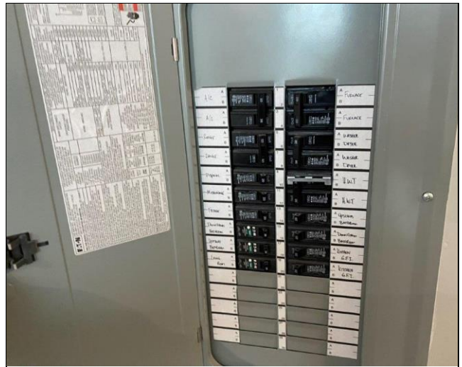
76. Typical dwelling unit breaker panel by Eaton
