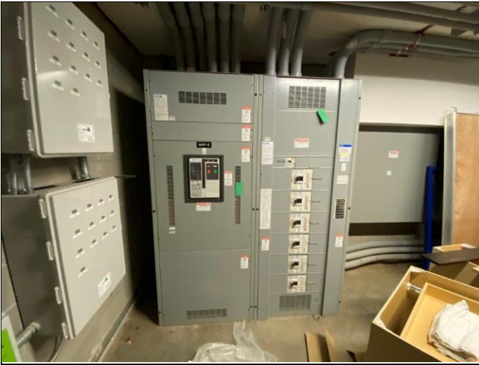
67. One of two electrical switchgear panels located in main electrical closet
