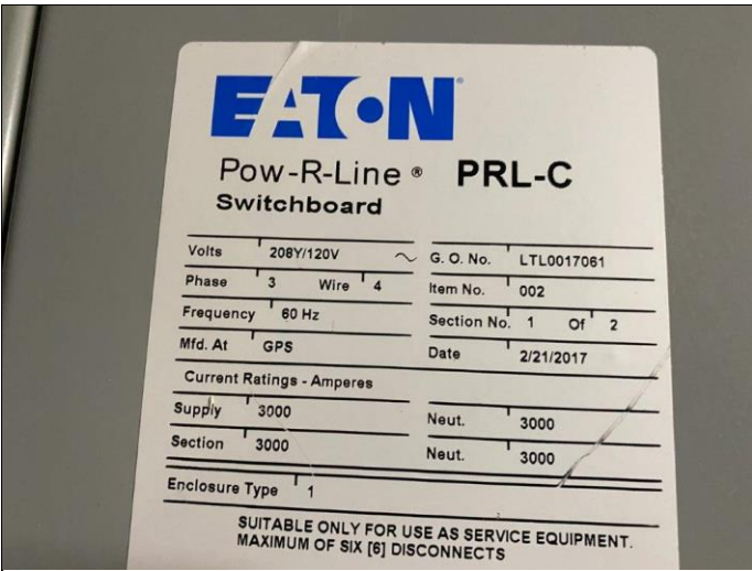
69. Switchgear label
