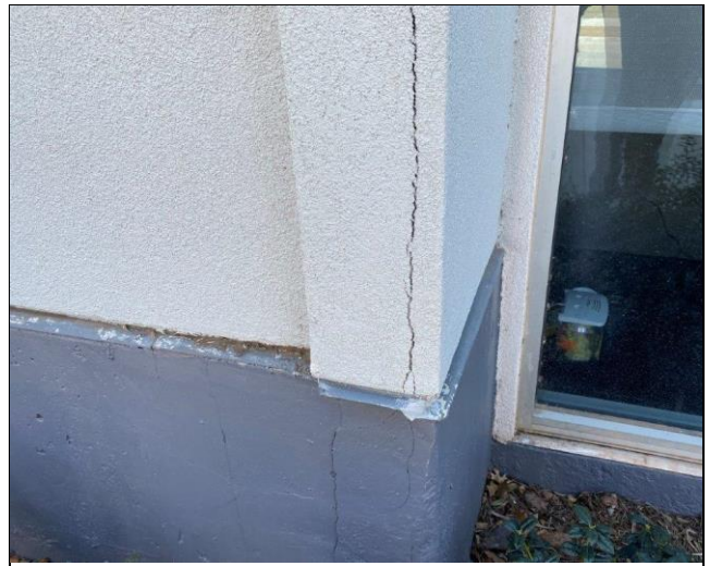
106. Cracking in the cementitious exterior finish system
