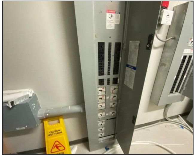
68. Typical electrical breaker panels and disconnects
