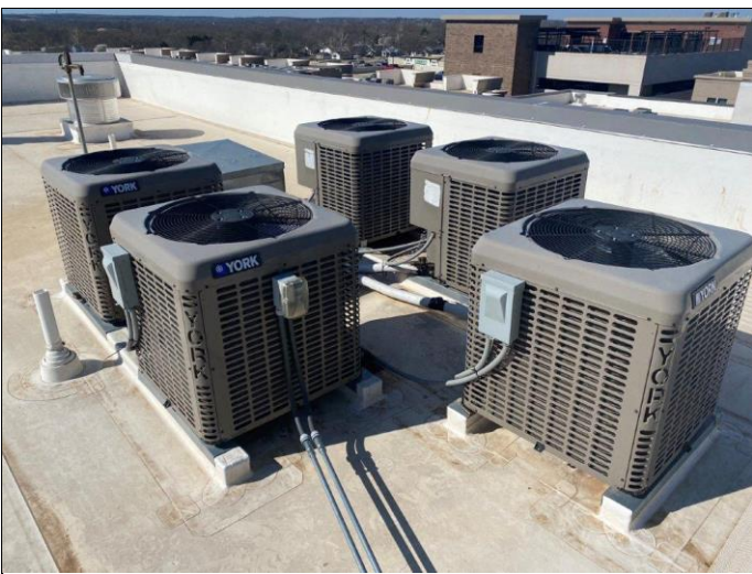
65. Typical split system condensing units at roof
