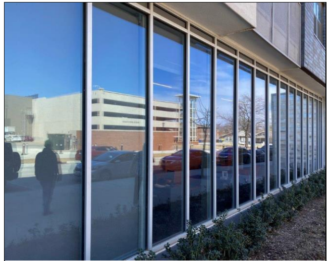
46. Curtain wall glazing system along the north façade
