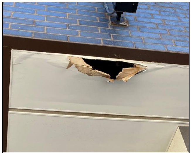
108. Water damage at an exterior soffit
