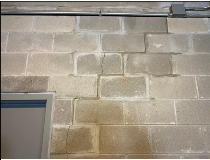
105. Linear and stepped cracking of load bearing CMU block walls at the bottom level
