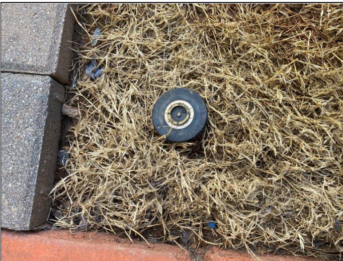
15. Typical irrigation sprinkler head
