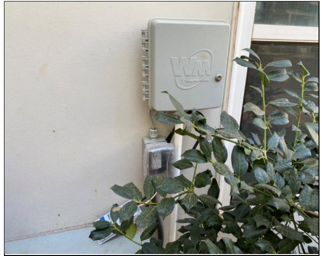
14. Automatic irrigation sprinkler system
