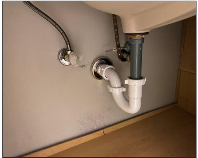
62. PVC sanitary sewer lines and vents
