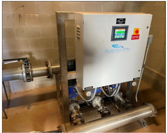
64. Water pump to boost water pressure located on ground floor accessed at south side of building
