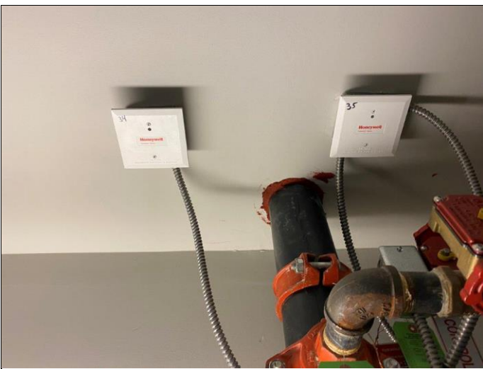
83. Electrical connections to flow alarms on fire riser
