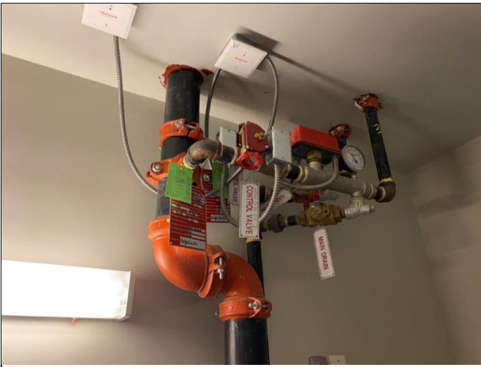
81. Typical fire riser located in stairwell
