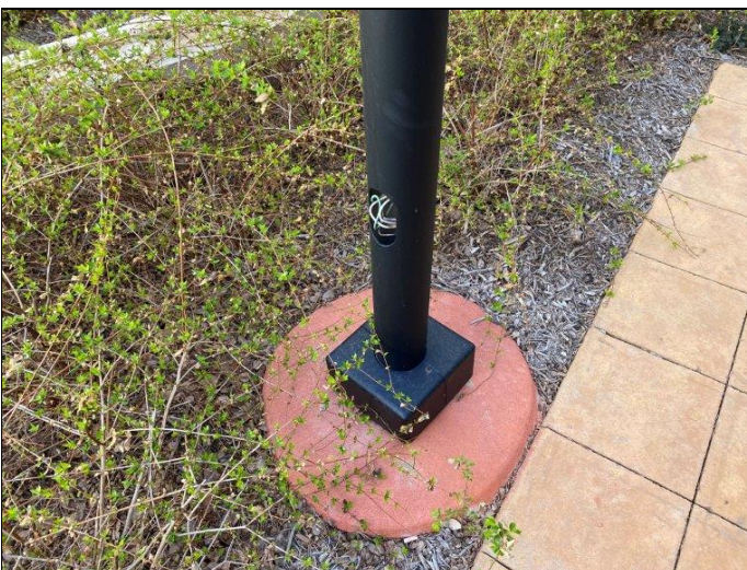
101. Missing electrical cover at light pole
