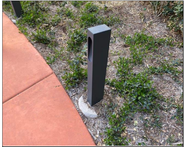
20. Bollard type light fixtures provided in the courtyard areas
