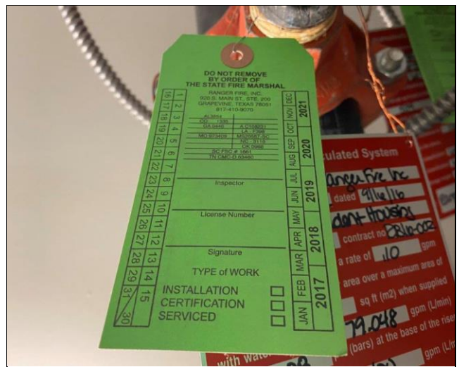
84. Fire riser inspection tags not filled out, typical
