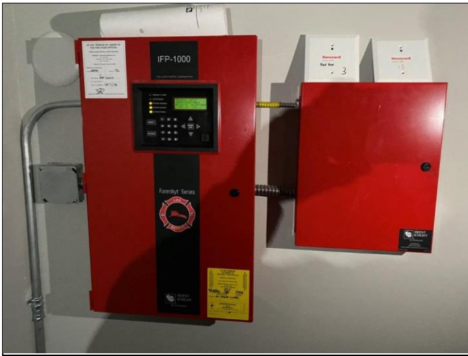
85. Fire alarm control panel (FACP)
