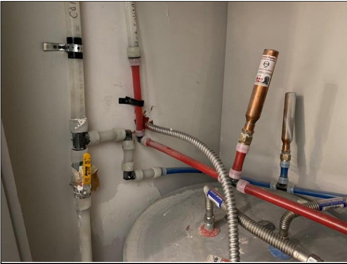
61. PEX water lines observed at water heater closet
