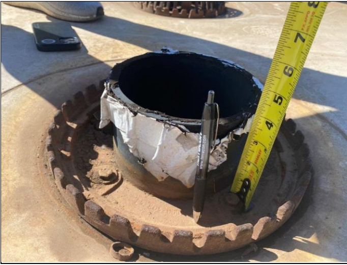
55. Emergency overflow drain measuring four inches above roof surface
