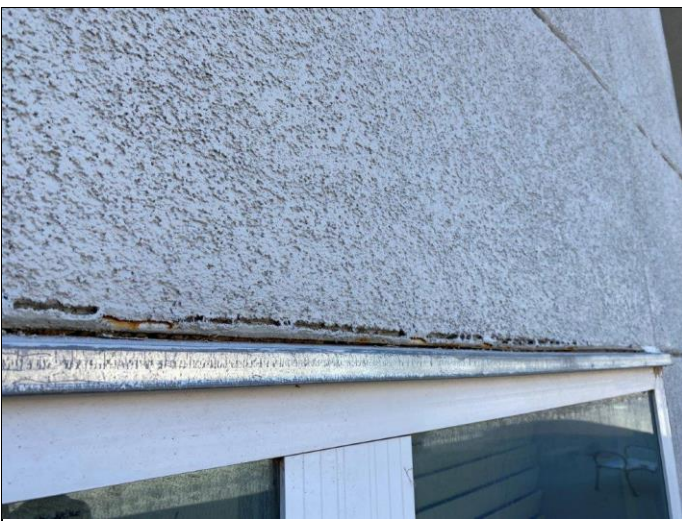
107. Cracking in the cementitious finish system above the dwelling unit windows
