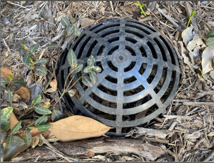
1. Typical stormwater drain in landscaped areas at internal courtyards
