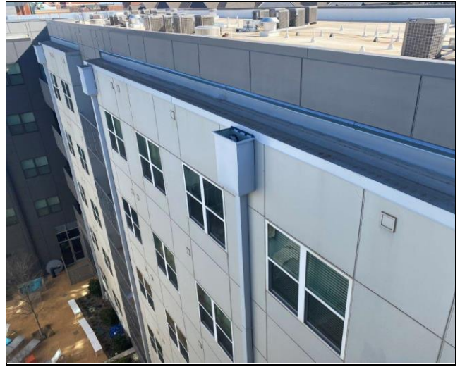
56. Bump out roofs drain to downspouts
