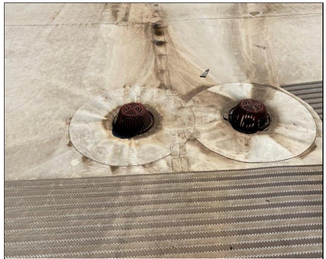
54. Typical internal roof drains
