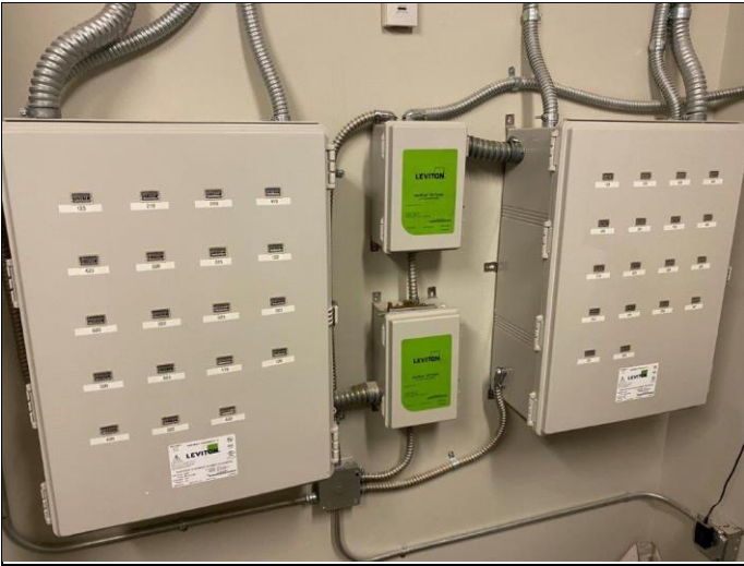
73. Unit electrical meters
