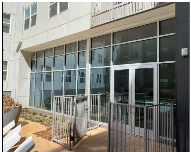
48. Curtain wall glazing system with integrated doors at the pool lounge area
