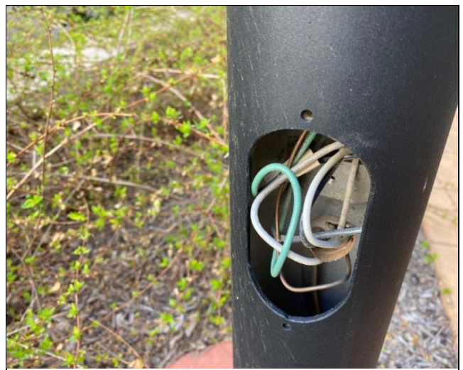
102. Missing electrical cover at light pole
