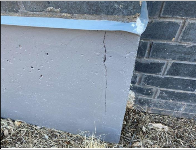
103. Cracking in foundation at the north side of the building
