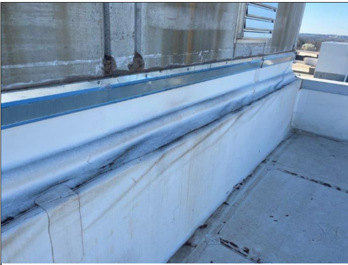
51. TPO membrane termination at concrete elevator shaft
